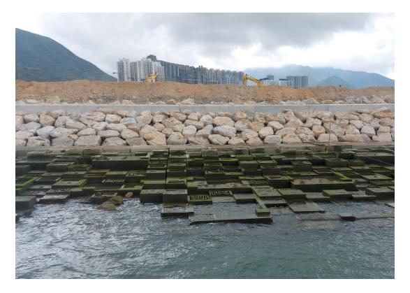
Photo 4 - Natural Rock Material/Planting for Artificial Seawall
